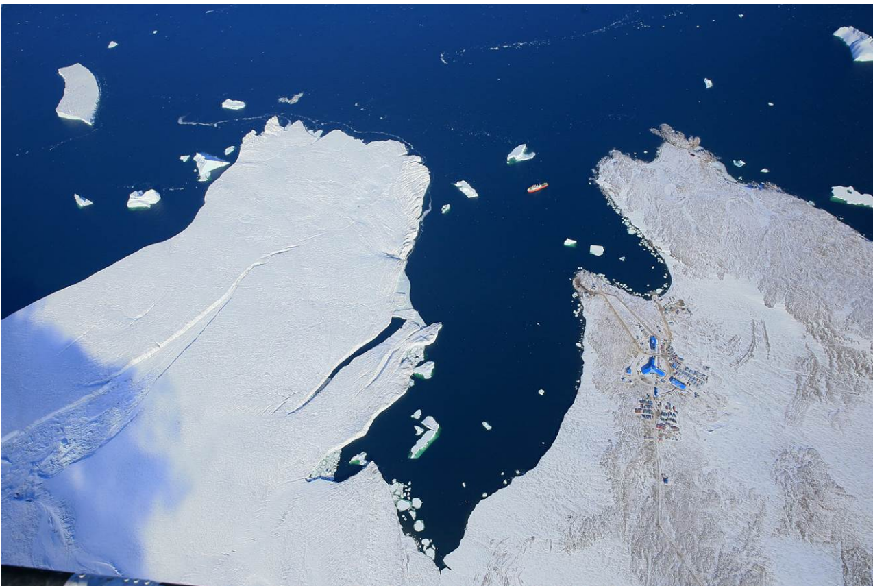
Figure 5: An Aerial view of the Jang Bogo Station before loading the construction camp containers
