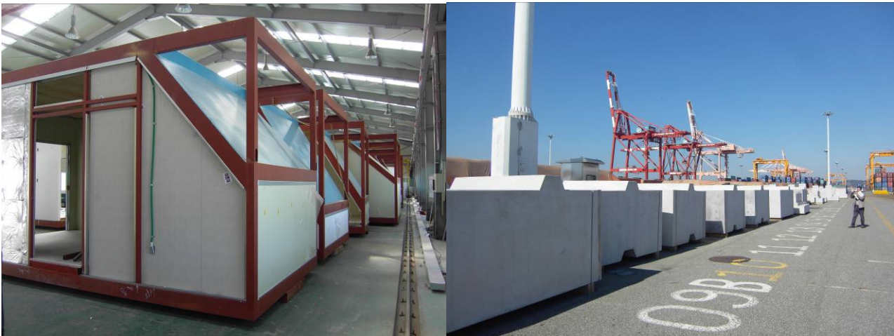
Figure 5: Modules for the main building and precast concrete foundations waiting for shipment
