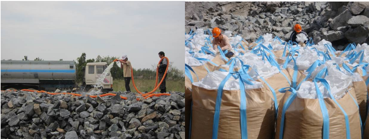
Figure 2: Cleaning and packing the riprap for pier foundation
