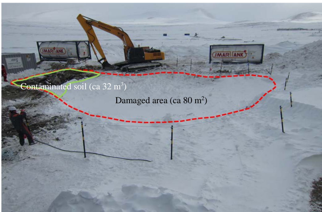
Figure 9: Damaged area with fence and about 32 m 3 of contaminated soil was removed.
