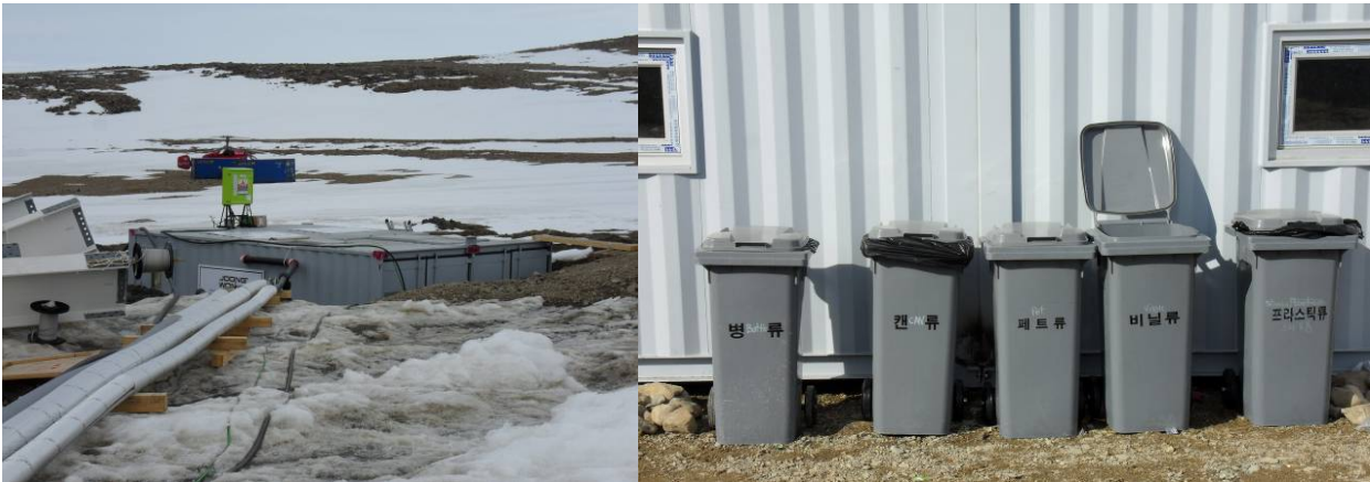
Figure 7: IC-SBR waste water treatment system and waste separation bins
