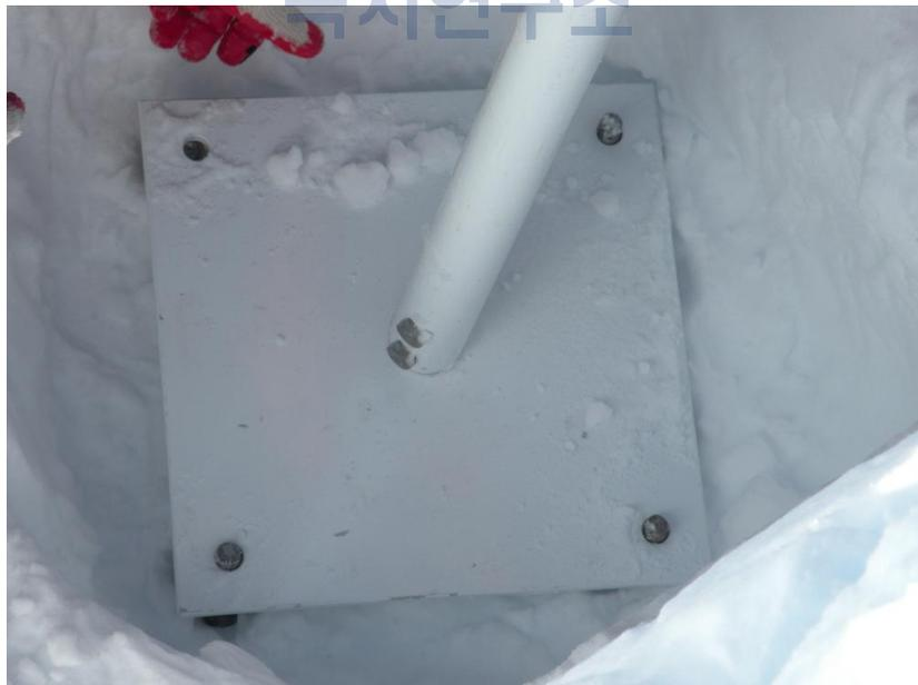
Figure 10.2: The base of the AWS tower in the hole
