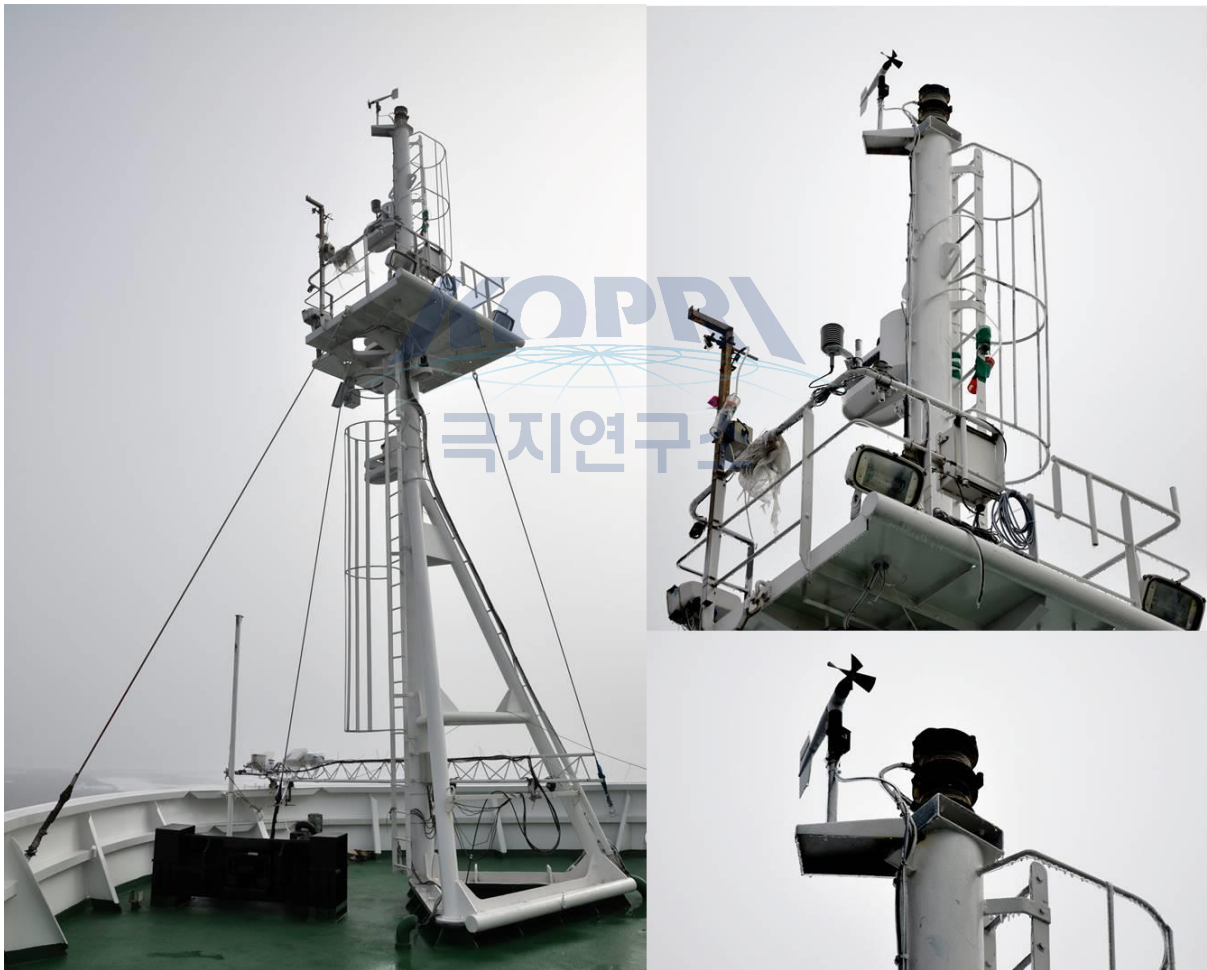
Fig. 1.2. Windmill anemometer at the foremast.
