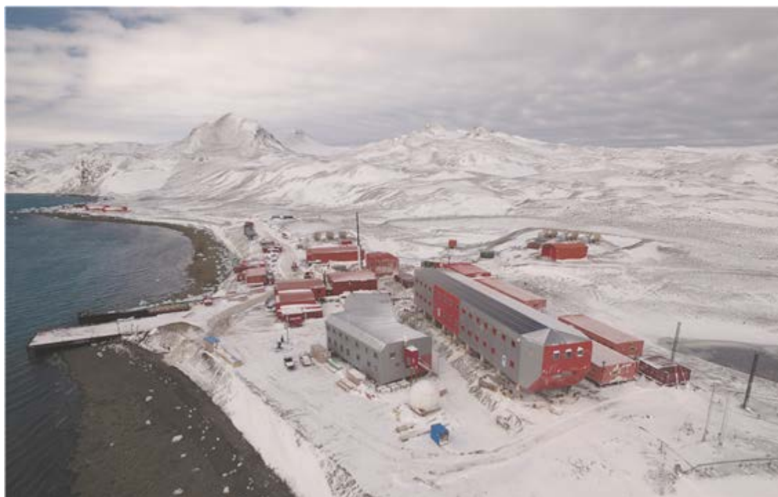
Figure 3. Aerial view of the King Sejong Station during the first renovation phase (on 1 March, 2017).
