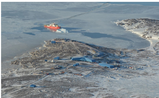
Fig. 1. Bird-eye view of Jang Bogo Station (courtesy of KOPRI).
