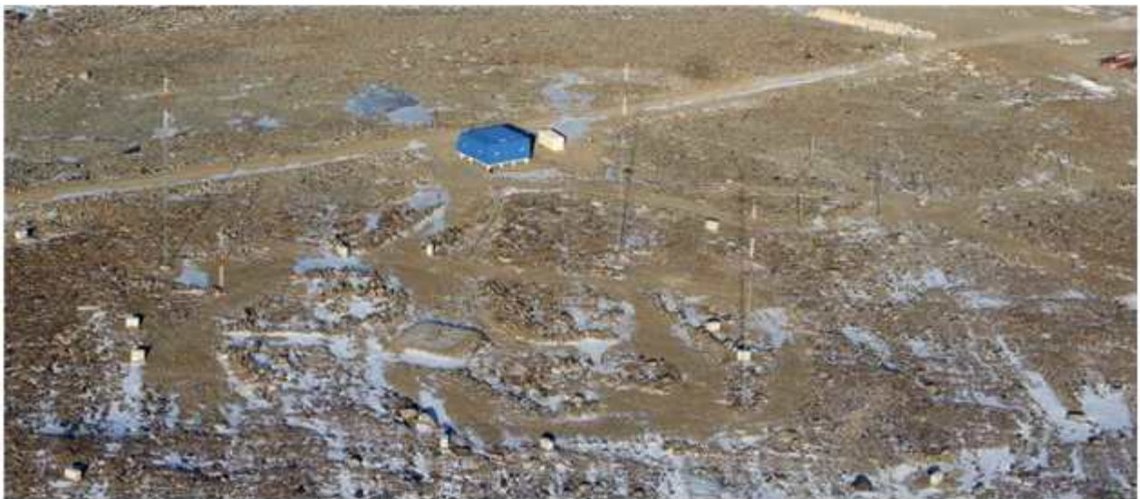
Fig. 30 Schematic diagram of VIPIR antenna array(top) and space weather observatory(SWO) and antenna towers(bottom).
