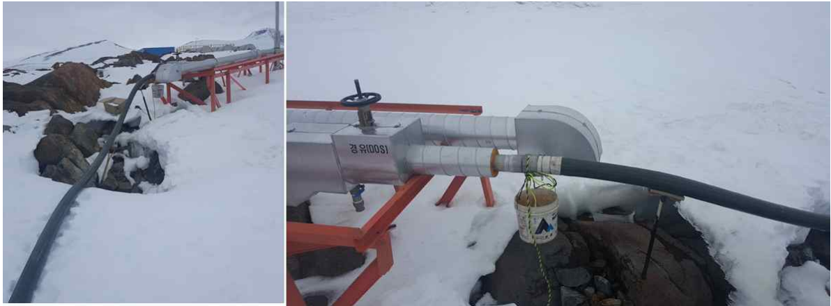
Fig. 1-14. Fuel transportation via hose with bucket in case of possible fuel spill at a joint.
