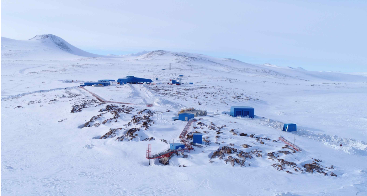
Fig. 2-1. Aerial view of Jang Bogo Station in 2017/18 early season.
