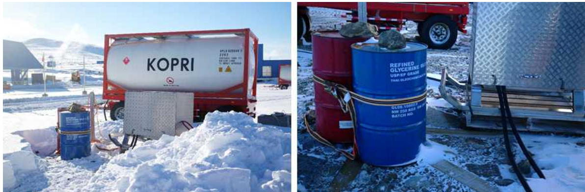
Fig. 9-4. ISO aviation fuel tank and service tank near by empty fuel drum to recover remaining fuel in the hose at Helipad.
