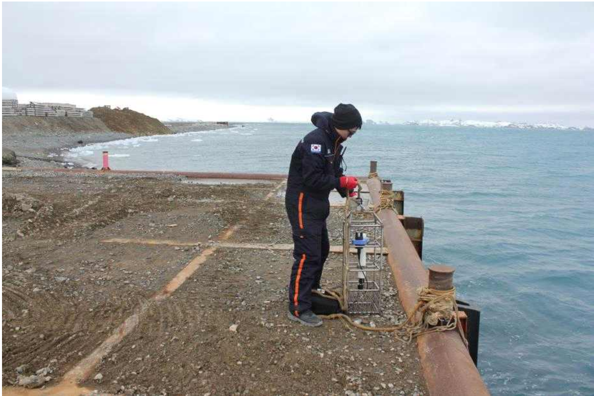
Fig. 7-6. CTD installation at dock.
