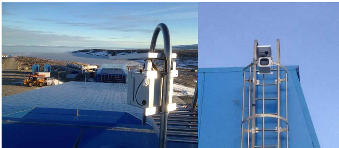
Fig. 4-15. Time-lapse camera for sea ice and cloud monitoring on the main building (left) and for snow-covered area change and cloud monitoring on the heavy vehicle storage (right).
