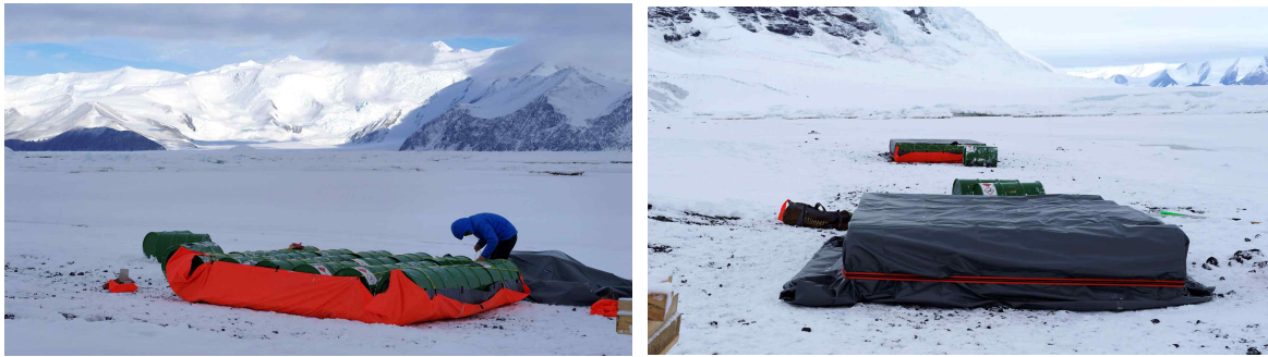
Fig. 2-7. Flexible bund to prevent fuel spill installed during 2017/18 season
