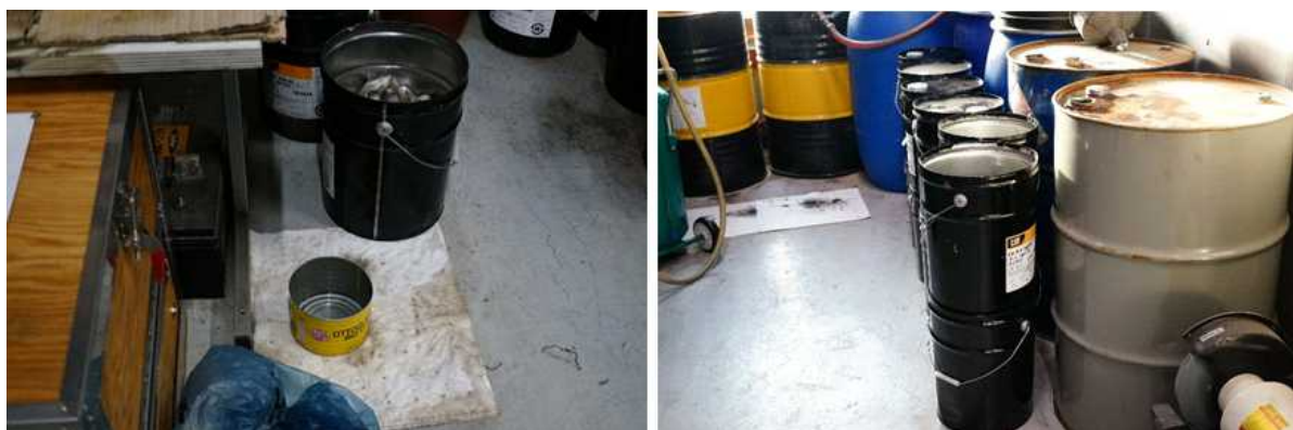
Fig. 9-5. Oil spill management in the power plant.
