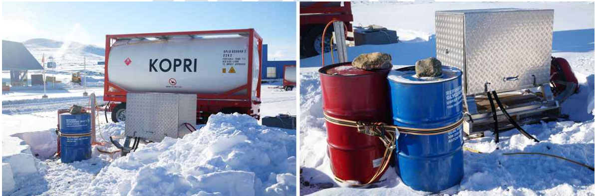
Fig. 1-15. ISO fuel tanks for aviation fuel(left) near helipad and waste fuel drum next by fuel service equipment(right).
