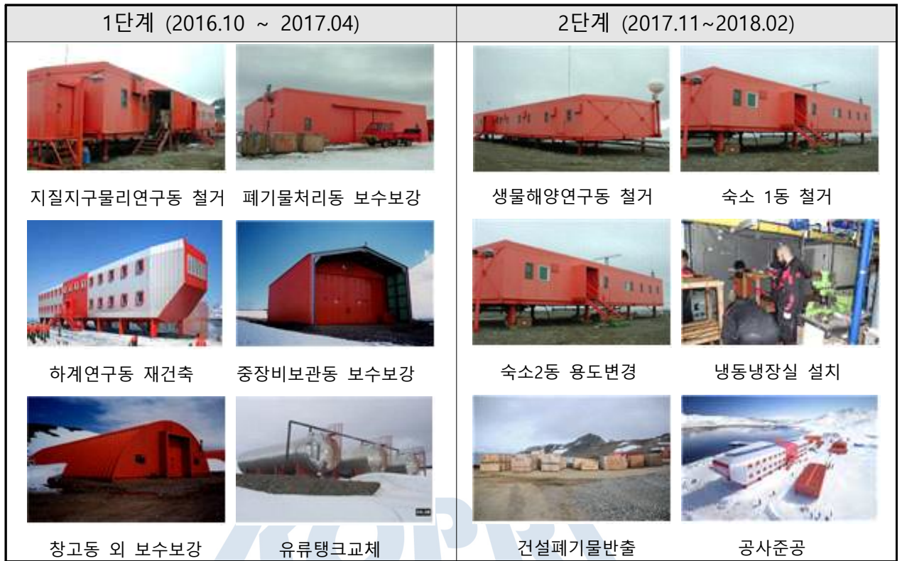
Fig. 6-2. Renovation works of King Sejong Station in 2016/17 and 2017/18 season.
