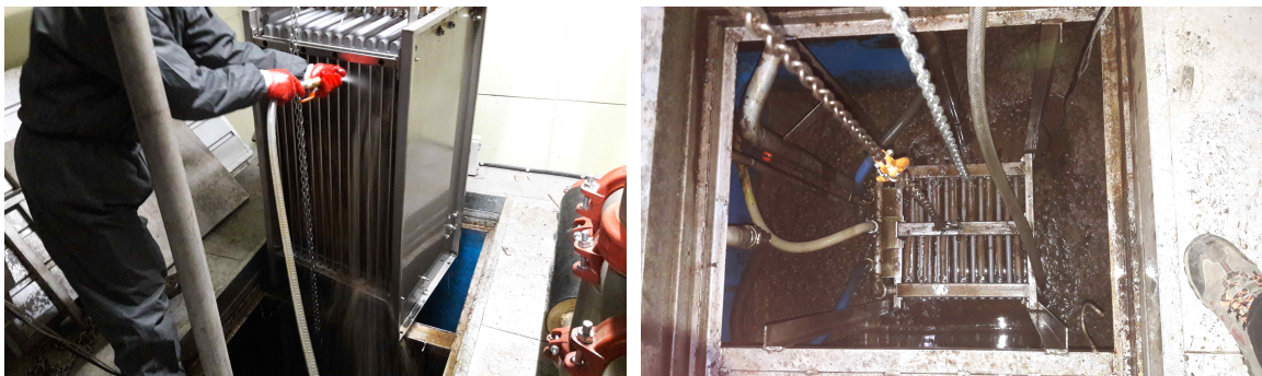
Fig. 1-1. Washing the membrane filter and reinstall to MBR module.
