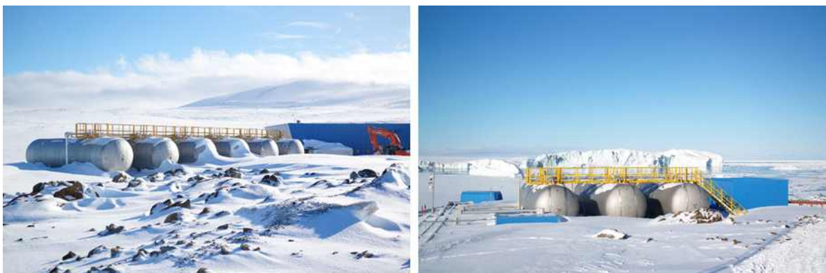
Fig. 9-3. Oil spill bund at Jang Bogo Station filled with snow due to heavy fall in 2017/18 season.
