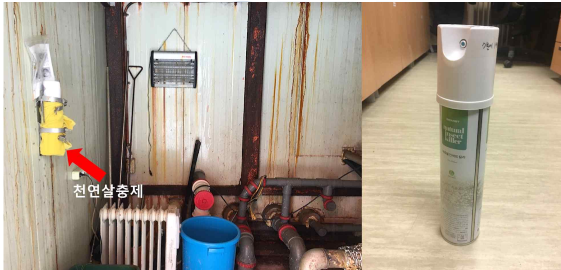
Fig. 7-4. Automatic spraying insecticide installed in sewage disposal plant (left) and natural spraying insecticide (right).
