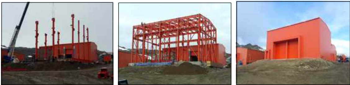
Fig. 6-2. New research boats storage house construction in 2018/19 season.
