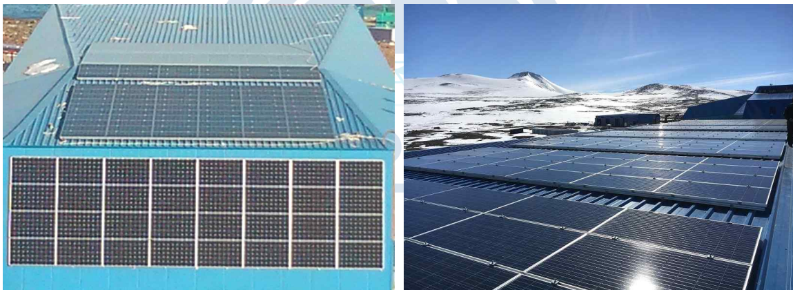
Fig. 1-14. Solar Voltaic Panels installed on Power Plants. existing panels (2014) and newly installed panels (2017).
