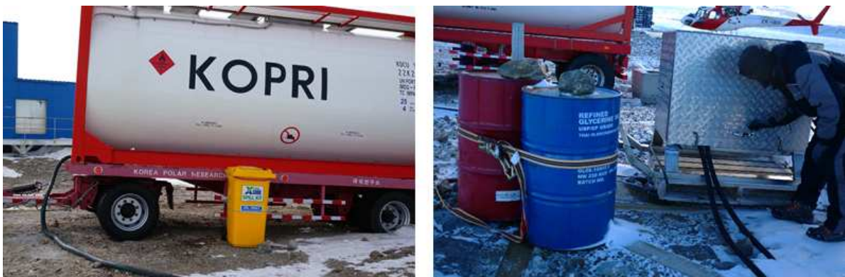
Fig. 1-13. ISO fuel tanks for aviation fuel next by spill kit (left) near helipad and waste fuel drum next by fuel service equipment(right).
