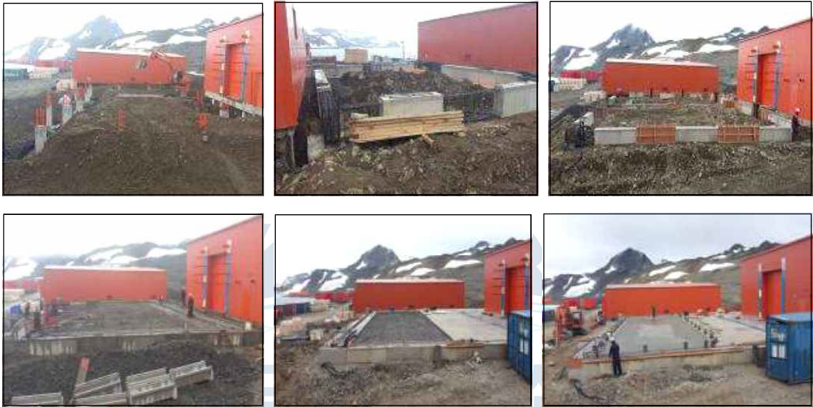
Fig. 6-1. Foundation works for new research boats storage house in 2018/19 season.
