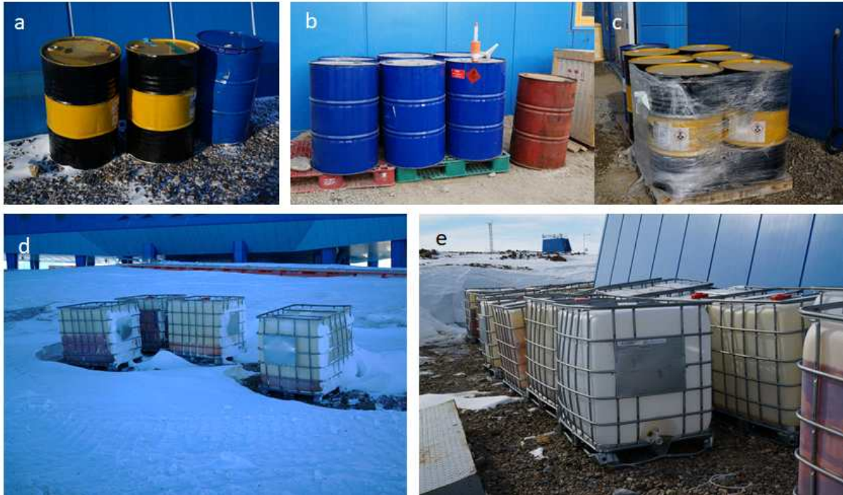
Fig. 9-4. Waste fuel and lubricant storage status at Jang Bogo Station. a. waste fuel drums on the ground in 2017/18 season, b, c. waster fuel drums on palettes in 2018/19. d. e. waste aviation fuel in plastic containers (d: 2017/18, e: 2018/19).
