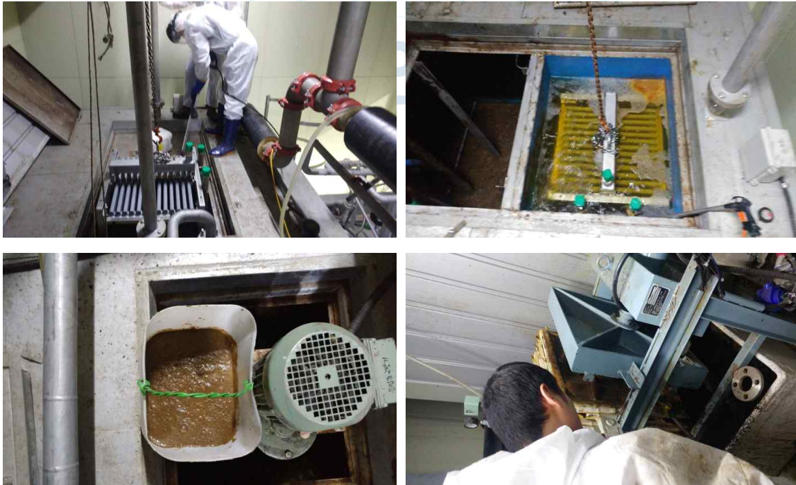
Fig. 1-1. Maintenance activities for wastewater treatment facility. washing the membrane filter and reinstall to MBR module (upper figures), sludge and remove water from sludge with presser (bottom figures).
