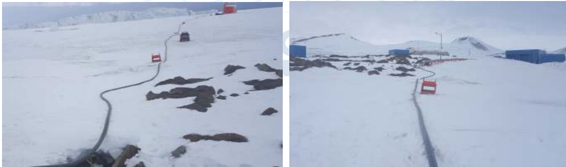
Fig. 1-11. Fuel transportation from ARAON to fuel tank in December 2017.
