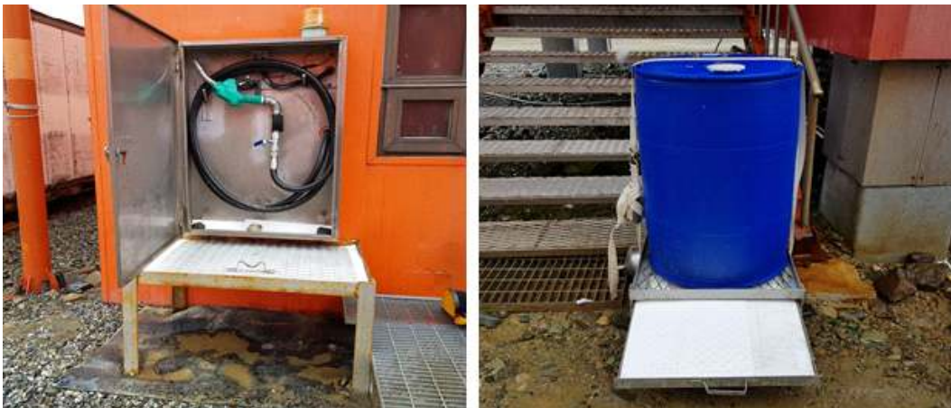
Fig. 6-10. Oil spill prevention measure for an oiler and for waste cooking oil tank.
