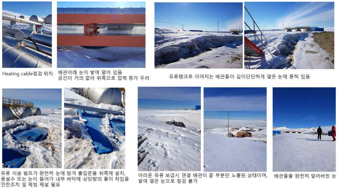
Fig. 1-3. Fuel supply pipelines and related facilities under heavy snow file cumulated for several 3-4 years.
