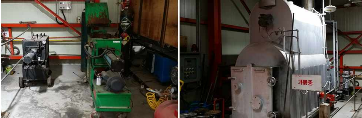
Fig. 6-4. Can presser and incinerator operating at King Sejong Station.
