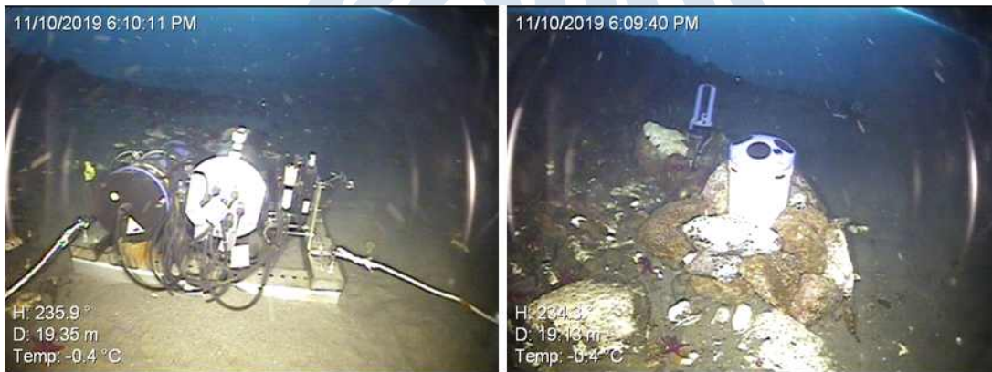
Fig 4-7. Reinstallation of bilogger and ADCP.
