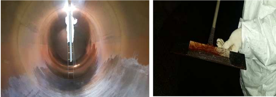
Fig. 6-8. Stain on the surface of inside of fuel tank.
