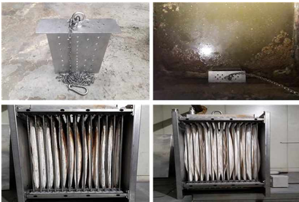
Fig. 2-1. Maintenance activities for wastewater treatment facility. Making and installing a screen filter to remove debris (upper figures), and replace MBR filter (lower figures).
