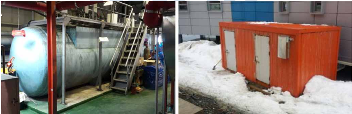
Fig. 6-3. Sewage inlet tanks installed in generator room (left) and next to accommodation building (right).
