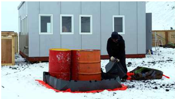
Fig. 1-5. Fuel spill prevention measures applied at Cape Hallett Camp in 2018/19 season.
