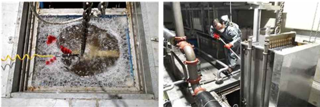
Fig. 2-2. Washing the MBR filter.
