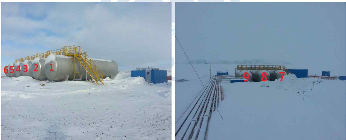
Fig. 2-10. Fuel storage tanks near power plant (No.1~6) and near dock (No.7~9)
