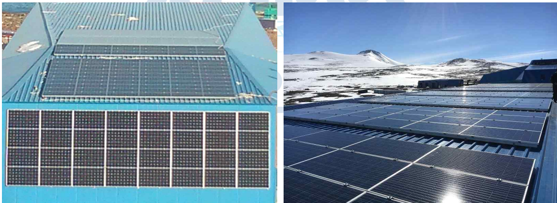
Fig. 2-14. Solar Voltaic Panels installed on Power Plants. existing panels (2014) and newly installed panels (2017).
