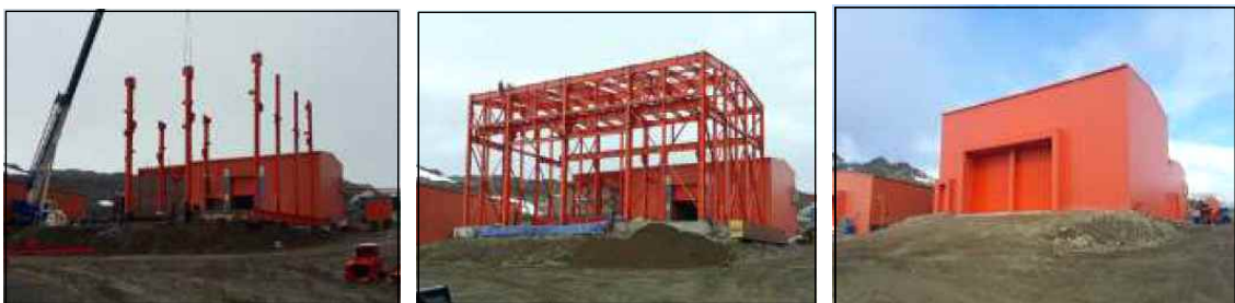
Fig. 7-2. New research boats storage house construction in 2018/19 season.
