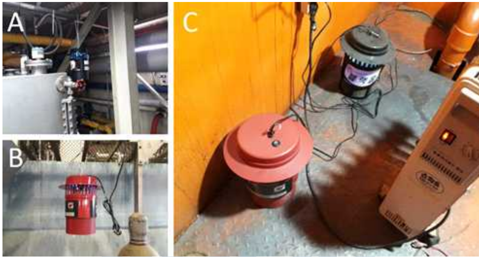
Fig. 8-3. UV traps installed in power building (A, B) and in sewage inlet building near accommodation building.
