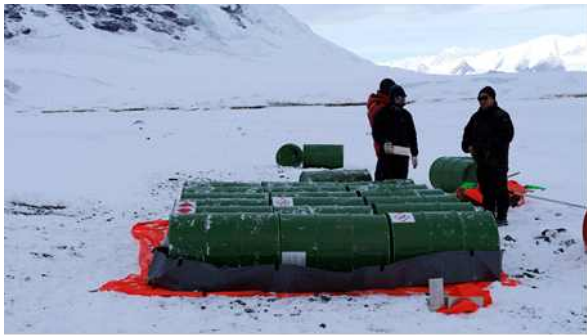
Fig. 1-4. A prevention measure for fuel spill (left), small amount of fuel spill from the valve of ISO aviation fuel tank (center and right)
