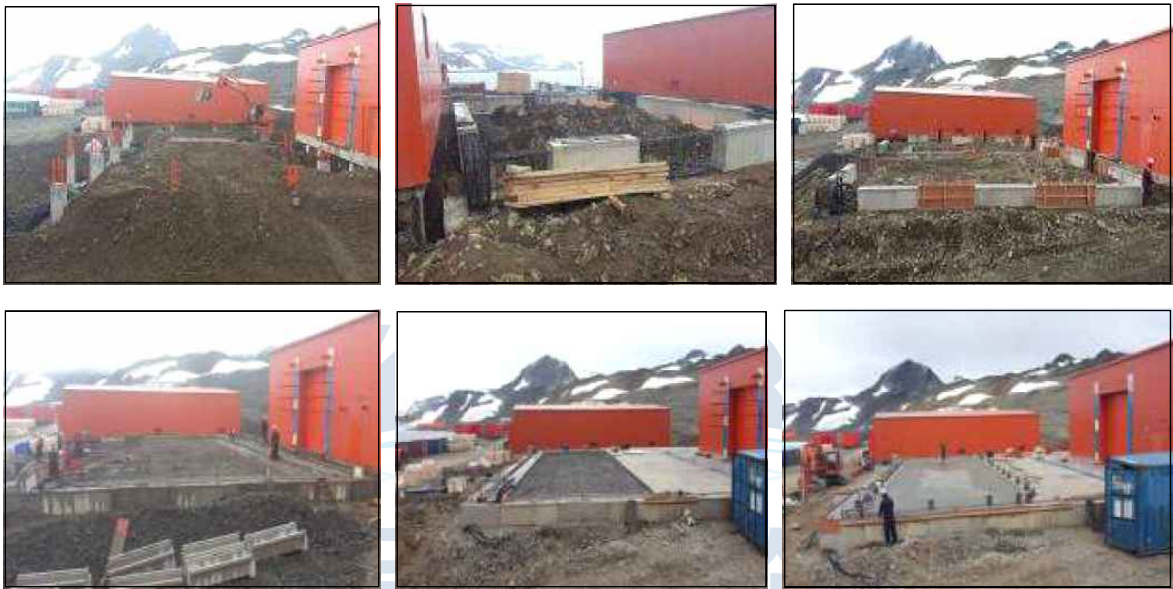
Fig. 7-1. Foundation works for new research boats storage house in 2018/19 season.
