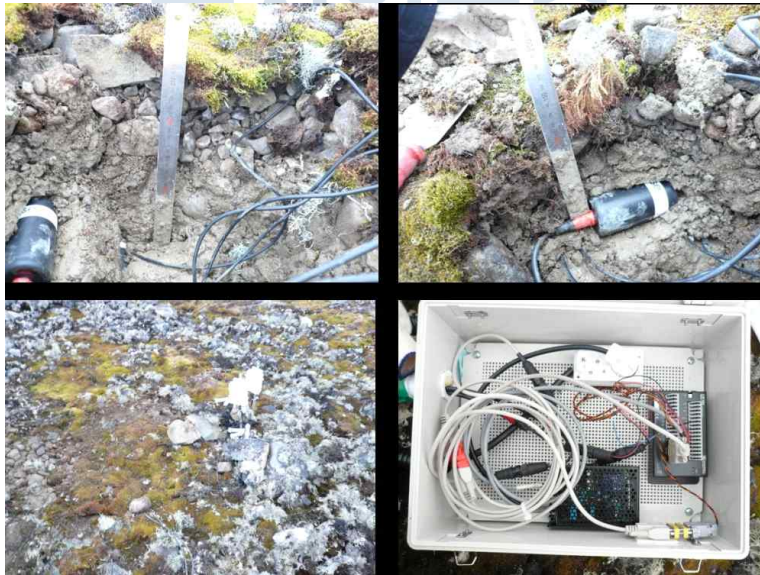
Figure 2. Installation of GP sensors into two soil layers and logging system.
