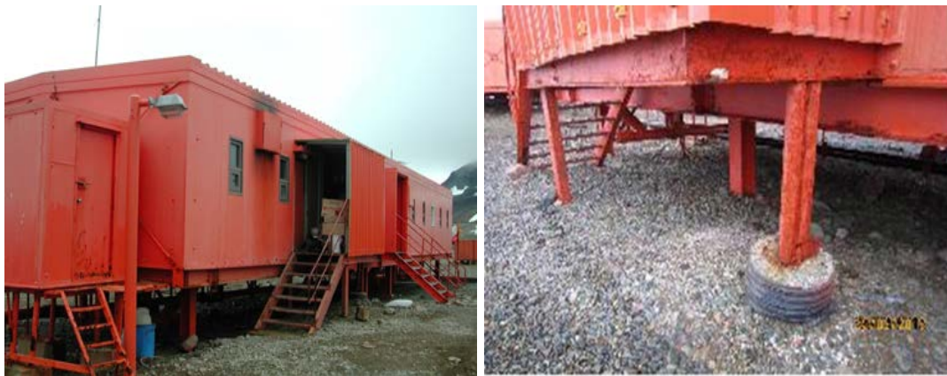
Figure 2. Current laboratory for geology and geophysics research (left) and its deteriorating foundation.
