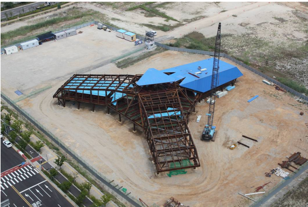
Figure 1: Pre-assembling of the main building of the Jang Bogo Station in Incheon, Korea
