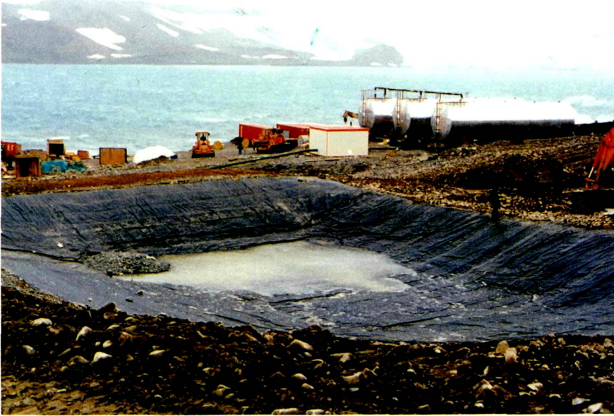
Fig. 7. Artificial lake "HYUNDAI-HD" with effective storage of 700m 3 .
