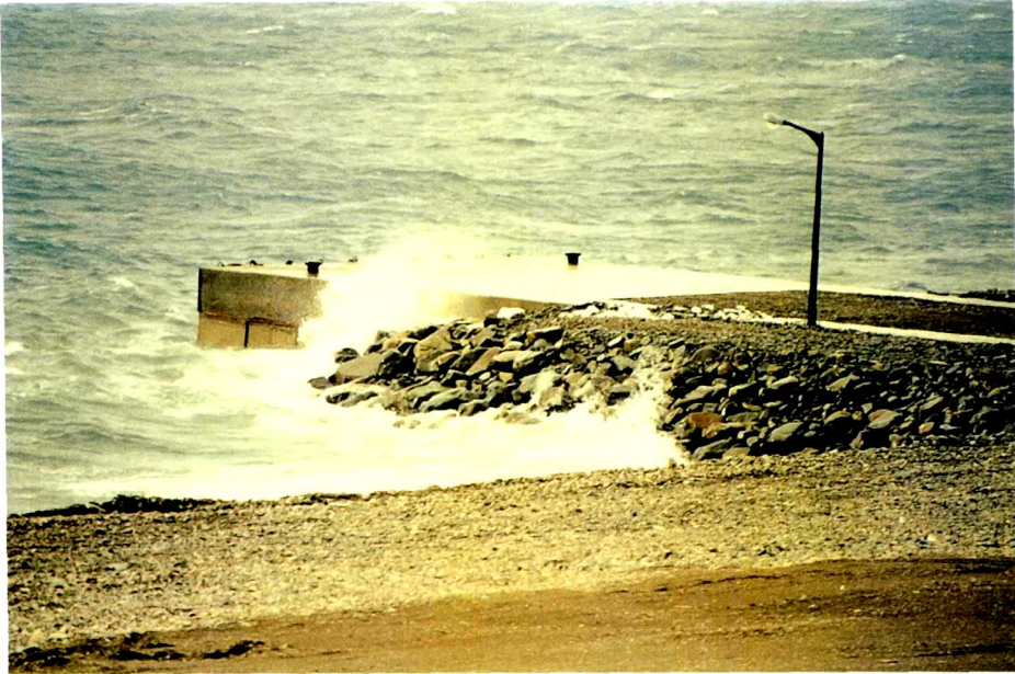
Fig. 6 . Concrete block type pier.
