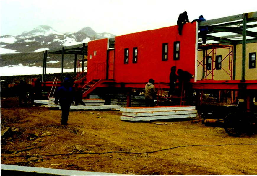
Fig. 5. Panel work for the main building.
